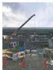
吊掛屋頂花棚
