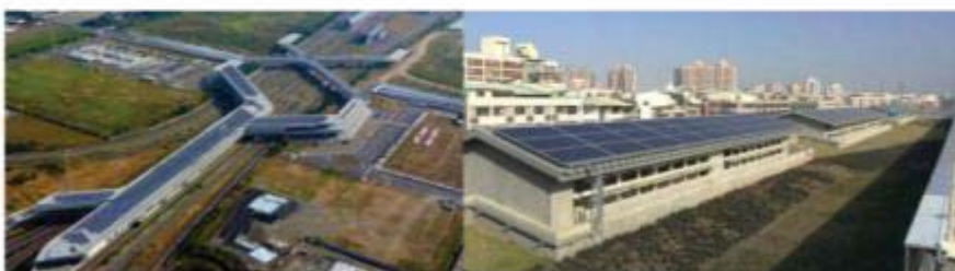
(b) Factories and traffic facilities
