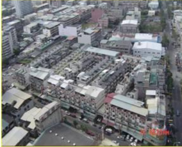
Iron Corrugated Roofs without Authorization
